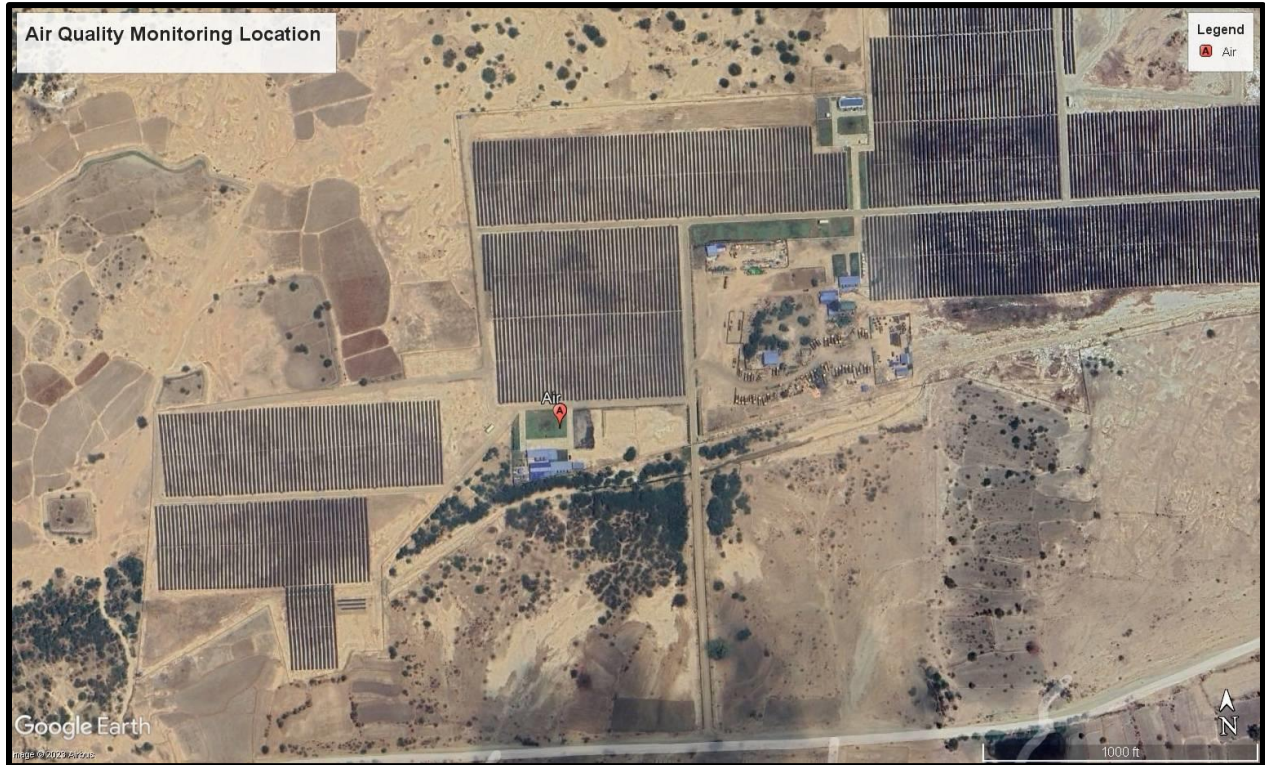
Figure 1. 2 Air Quality Monitoring Locations of Thapyaywa Solar Power Project
